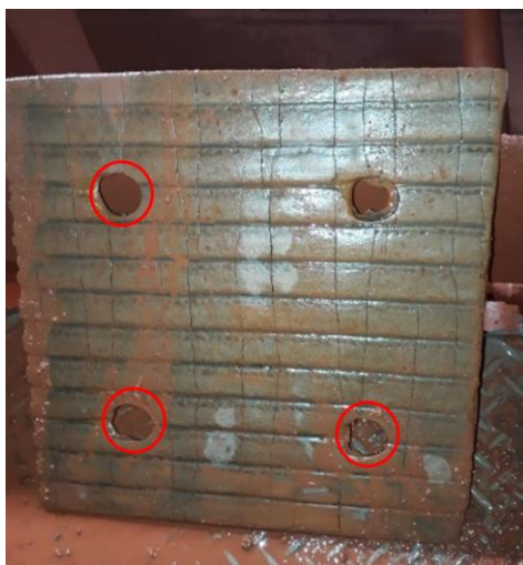
Figura 31. Chapa desprendida do chute Over da Peneira 631B-PV-0005
