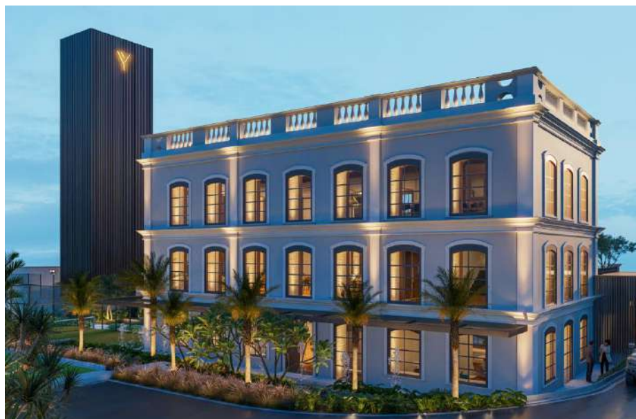
Figura 06 – fachada Palacete Camelier
