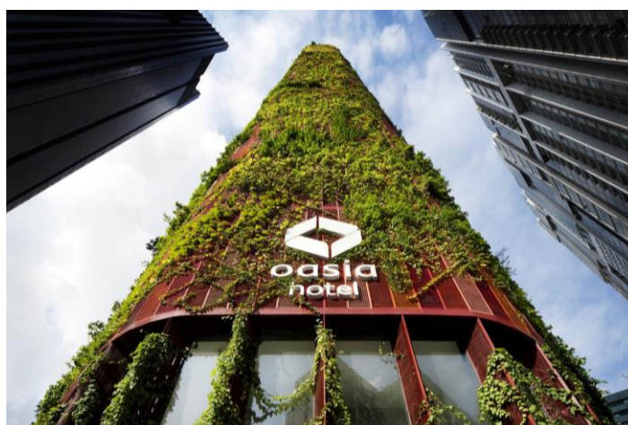
Figura 08: Fachada frontal do Hotel Oasia Downtown.
